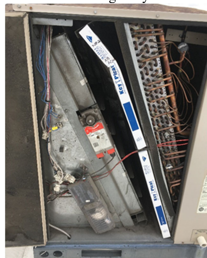
Figure 4. Picture of a filter that is not seated correctly.
