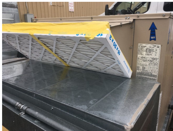
Figures 6-a and 6-b. Picture of a MERV 13 filter installed on an outdoor air intake as supplemental filtration
