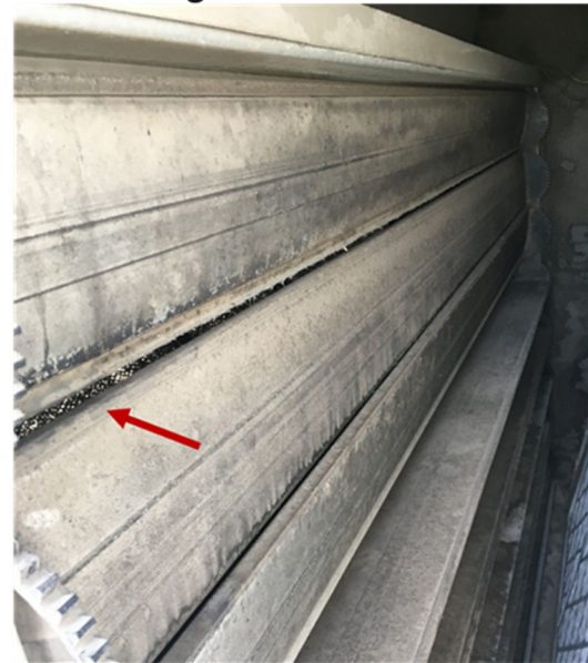
Figure 3. Picture of a warped damper blade unable to close.
