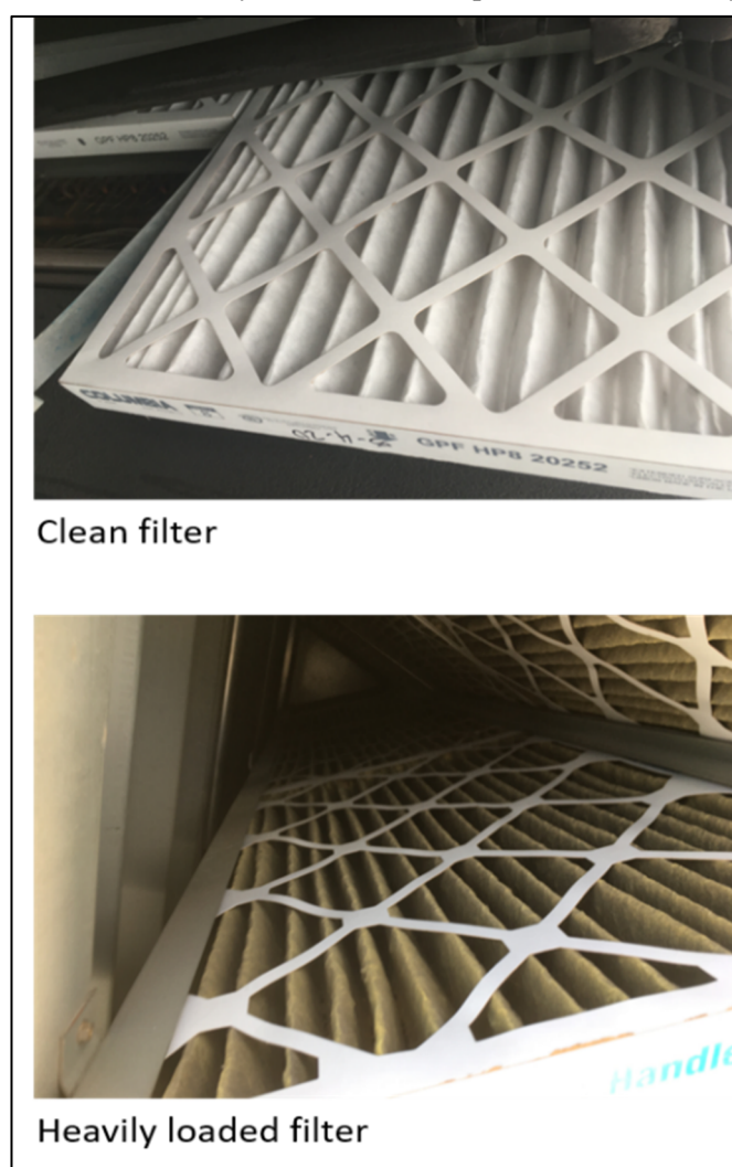
Figure 5. Comparison of a clean filter to a filter heavily loaded with wildfire smoke.
