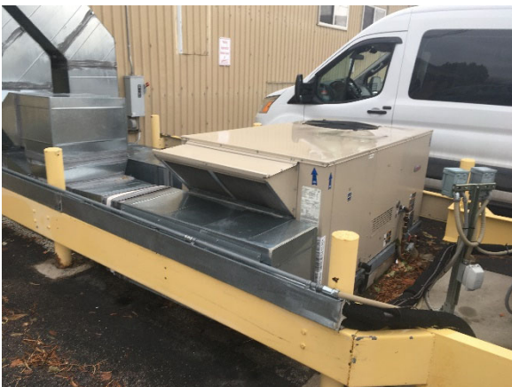
Figures 6-a and 6-b. Picture of a MERV 13 filter installed on an outdoor air intake as supplemental filtration
